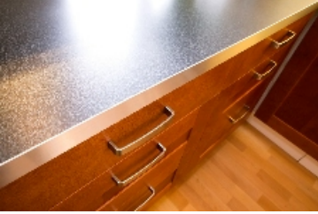
The heat resistant nature of thermoset plastics make them ideal for kitchen surfaces. The plastic is applied as a veneer to a chipboard core.
